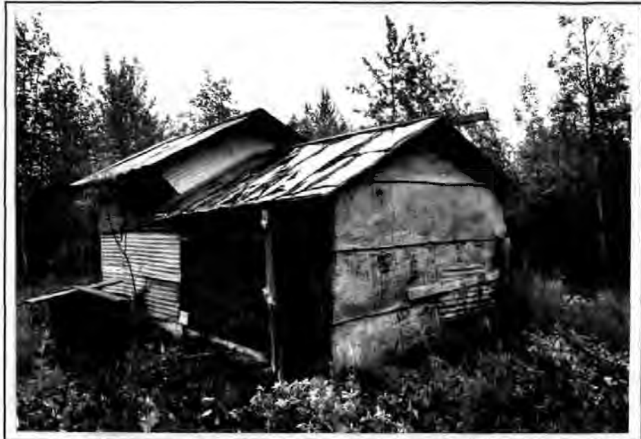
Figure 122. The Parker/Flemings Meat Shed, 1993. The view is looking southeast.
